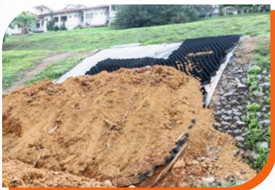
Erosion Control & Slope Protection
