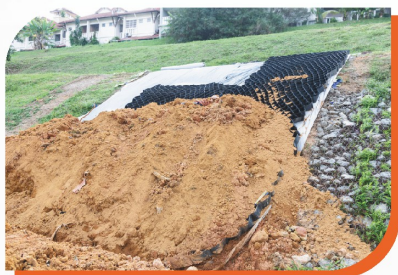
Erosion Control & Slope Protection
